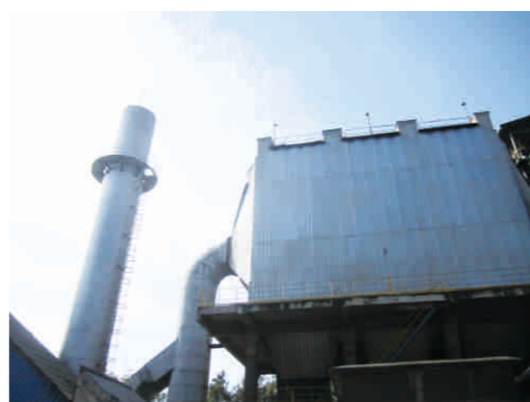
华新（宜昌）公司加强工艺控制，提高电收尘效率，窑头粉尘排放浓度稳定控制在30mg/m 3 以下。 Huaxin (Yichang) Co. enhances process control, improve filter efficiency, kiln head dust emission thickness is controlled under 30mg/m 3 .
