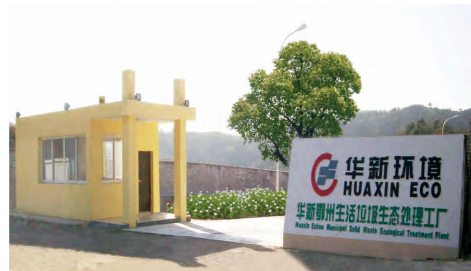
华新鄂州生活垃圾生态处理工厂大门 The gate of Huaxin Ezhou Municipal Solid Waste Ecological Treatment Plant
